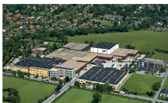
NORD DRIVESYSTEMS, Headquarters Bargteheide
