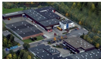
NORD gear factory Glinde
