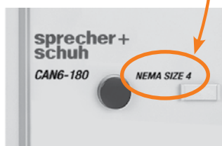
CAN6 NEMA labeled contactor (AC)
